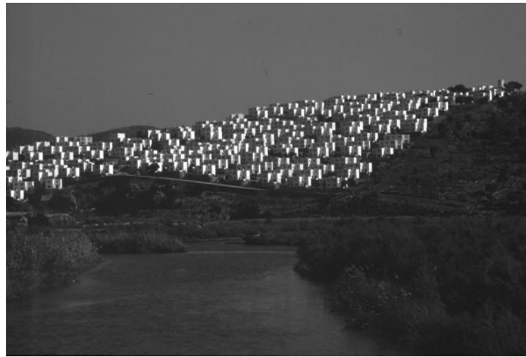
Illegal buildings on Salaman coast, Turkey. Tourism development is in direct competition with other forms of land-use (agriculture, nature conservation).
